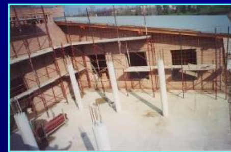
Pilastri e travi in c.a.
